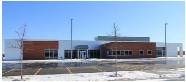
Emergency Management Training Center (EMTC) for classroom (location 6-78 on Cantonment Map)
